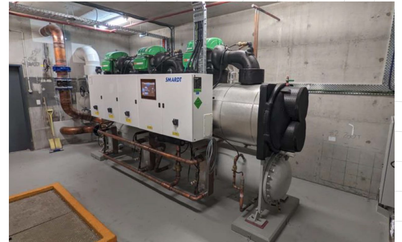
The recently installed Smardt Powerpax chiller
